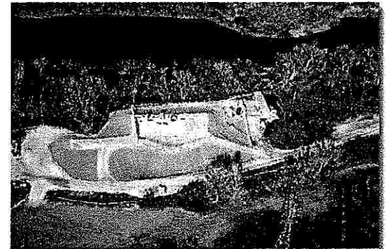
SRWA Pump Station
