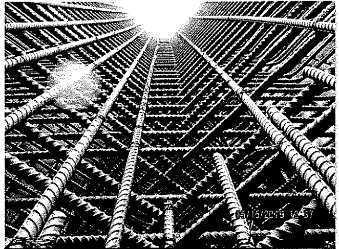
Pump Station Reinforcing Steel
