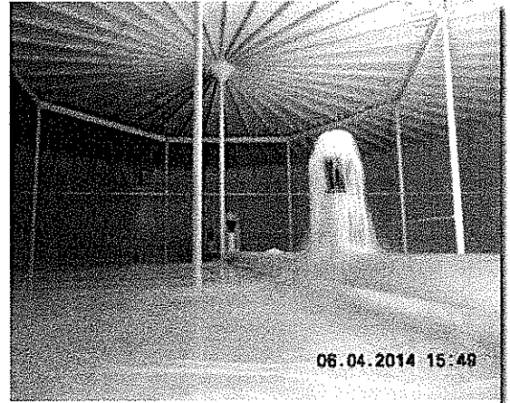
Potable Water Tank
