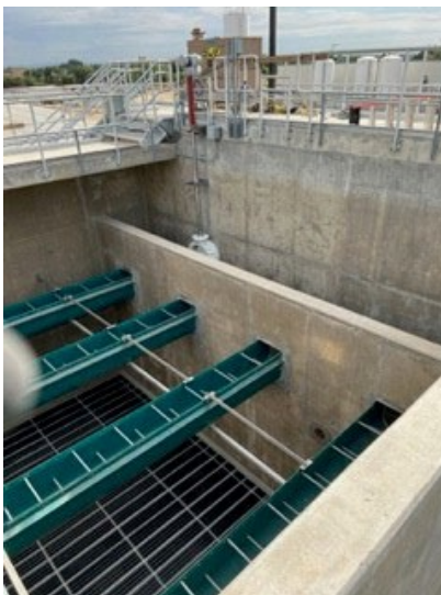
figure 3 - Filter Underdrain
