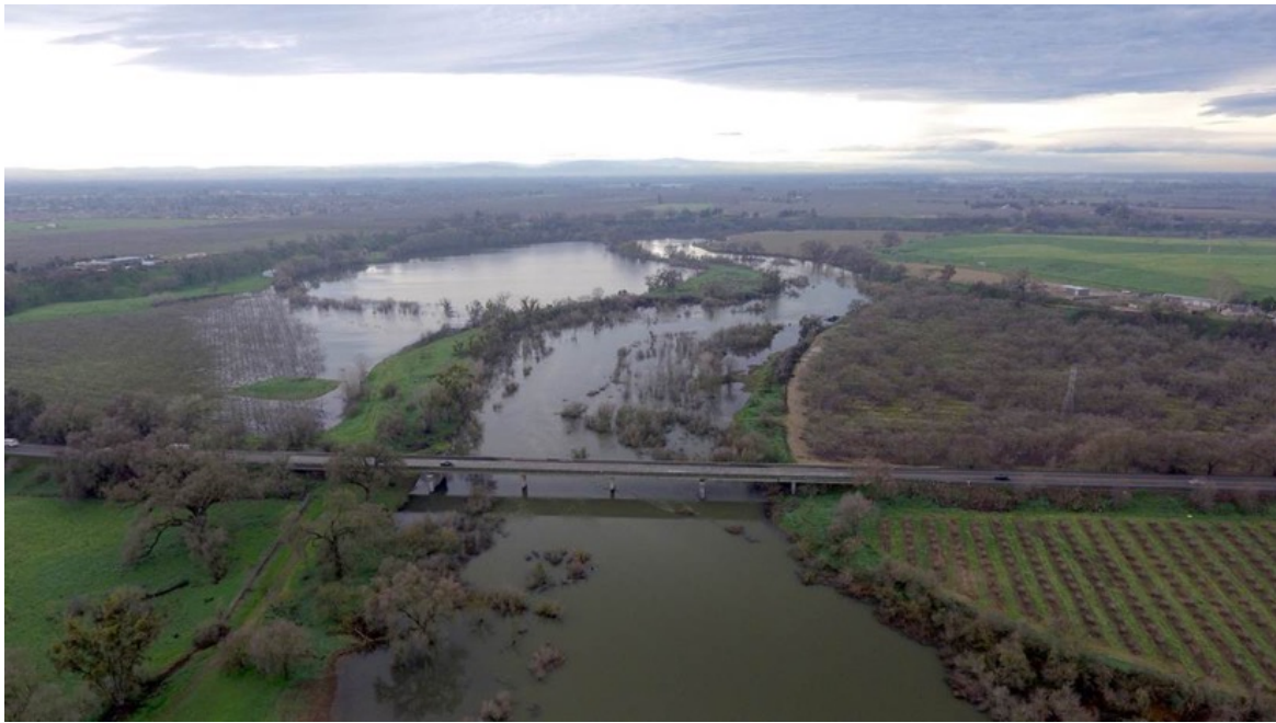
Figure 4-1. Photo of flooded Tuolumne River near infiltration gallery and source water sampling location, January 5, 2017
